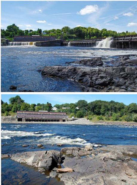
**Fig. 4.** Veazie Dam, one of two downstream dams on the Penobscot River in Maine, USA, was removed in 2013 as part of a basin-wide settlement agreement among stakeholders. Before (top) and after (bottom) photographs taken by Josh Royte of the Nature Conservancy (used with permission).
